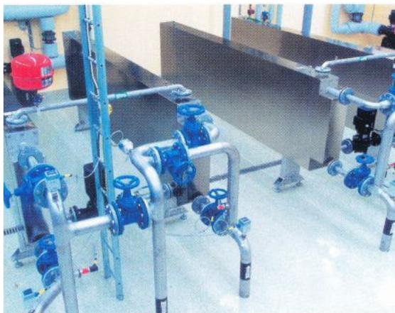
Two heat exchanger units sludge/sludge installed at Vimmerby wastewater treatment works in Sweden
