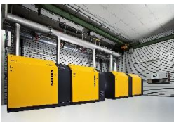
Modern rotary screw blowers can be arranged side-by-side
